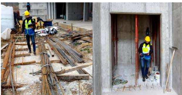
Figure 4. Mapping the construction site with the iMMS.
