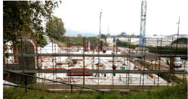
Figure 2. Construction site as of 19/10/2021.
